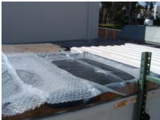
Fig. 3: Two variations of the solar puddle under construction.
